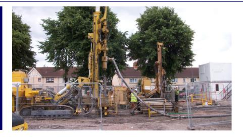
The scheme involved installation of a grid of boreholes for a closed loop Ground Source Heating system to a primary school extension in Walsall. 15 nr 150mm diameter boreholes were drilled to 100m depth through 9m of overlying loose fills and then through coal measures strata including worked coal seams which were infilled and grouted as drilling progressed.
